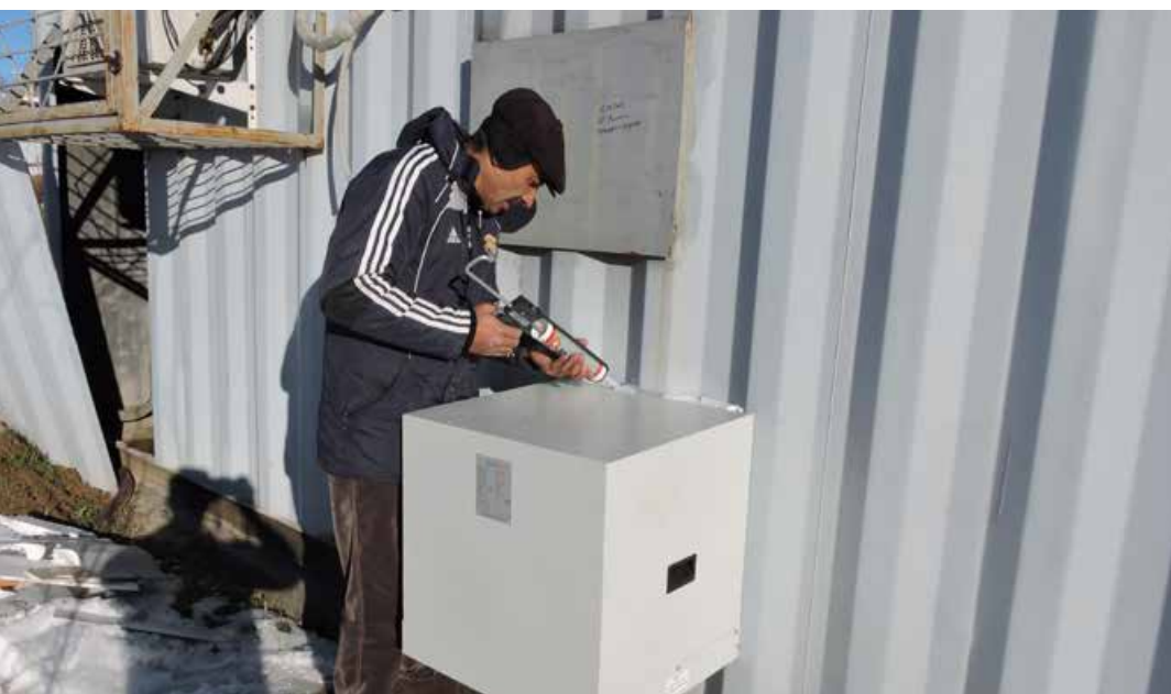
INSTALLATION OF THE ENERGY EFFICIENT COOLING MODULE AT MOBILE BASE STATION. PHOTO CREDIT: UNDP TAJIKISTAN
