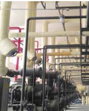
WORKSHOP OF CHINA'S LARGEST NH 3 /CO 2 REFRIGERATION SYSTEM WITH 16 SETS EACH OF NH 3 AND CO 2 COMPRESSORS. PHOTO CREDIT: YANTAI MOON GROUP CO. LTD.
