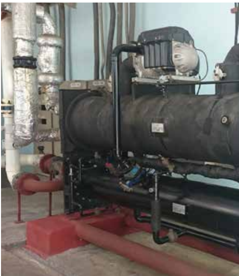
OLD AND NEW CHILLERS AT SANTA CLARA HOSPITAL. PHOTO CREDIT: CARLOS ANDRÉS HERNÁNDEZ, UNDP MPU
