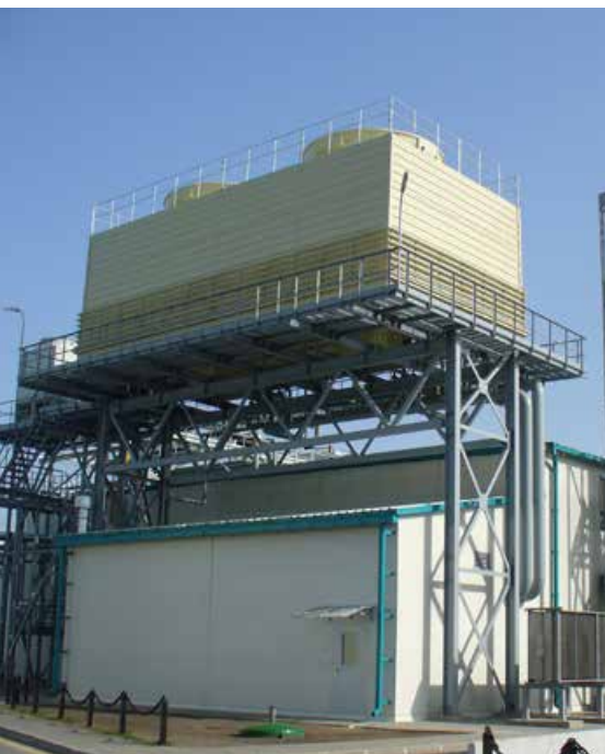
GENERAL VIEW OF ENERGY COMPLEX “SANTA BREMOR” IN BREST, BELARUS. PHOTO CREDIT: VALERY PISHCHIK
