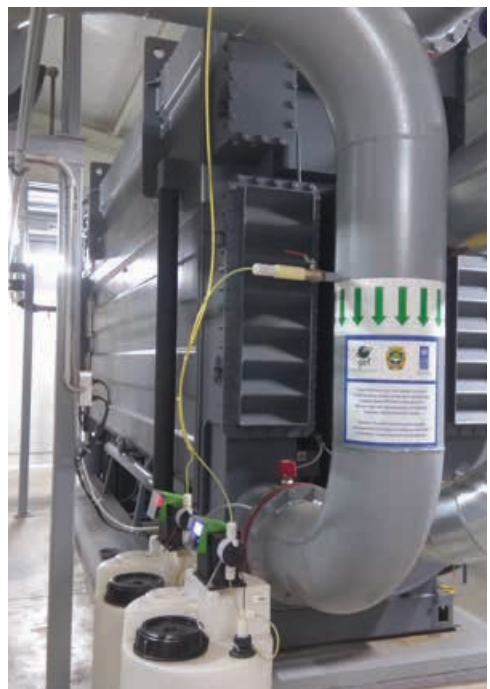
ABSORPTION REFRIGERATING MACHINE (ARM) – HEART OF THE ENERGY COMPLEX. PHOTO CREDIT: VALERY PISHCHIK
