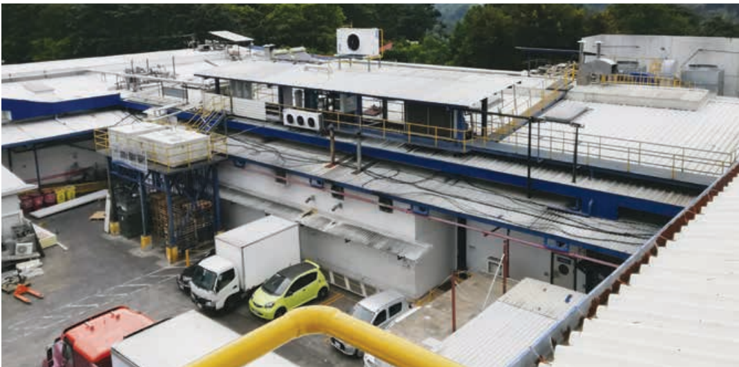
GENERAL VIEW OF THE FACTORY FROM THE PLATFORM WHERE THE EQUIPMENT WILL BE INSTALLED. PHOTO CREDIT: RODOLFO ELIZONDO
