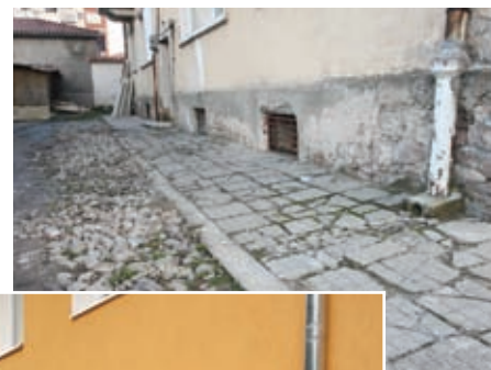
Restoring pavements and updating drainage systems protects the building foundation: before (top) and after (below). UNDP Bulgaria
